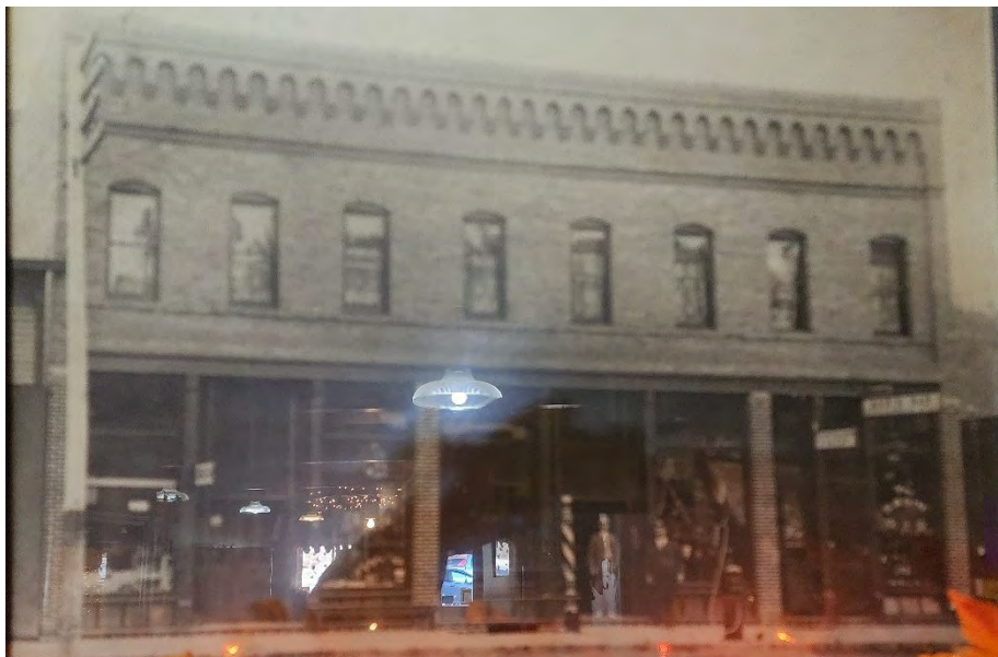
The Silver Saddle Bar and Café probably closer to its 1885 construction date.
