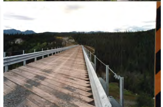
An Alaska trip side trip. A rail road bridge to an abandon Endecott Copper Company mine, converted to a vehicle roadway.
