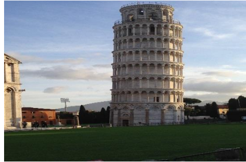
Yes, it does lean as do all the other buildings around it.
