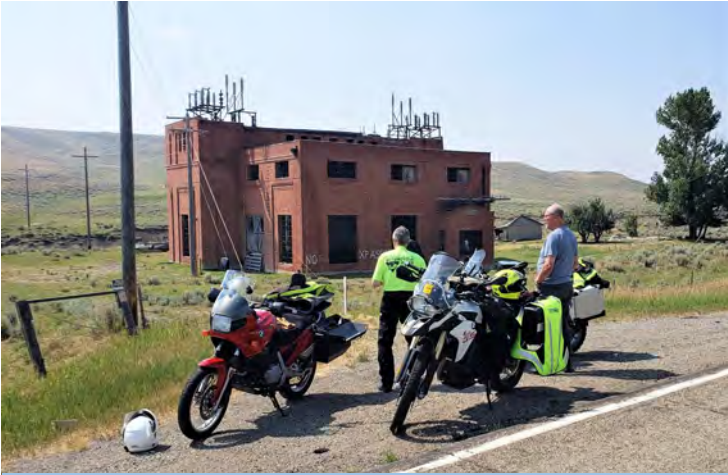
Abandon Milwaukee Railroad substation (Substation No. 2) at Loweth, Montana about 47 miles west of Harlowton, the start of the electrified segment which ended in Avery, Idaho. Ken Conrad and Dean Hall in the photo.
